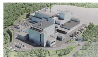
Volume reduction facility in Futaba Town, Fukushima Prefecture
