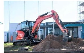
Example of investment for production increase : Hirakata plant
