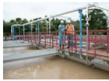
Constructed water treatment facilities in Myanmar
