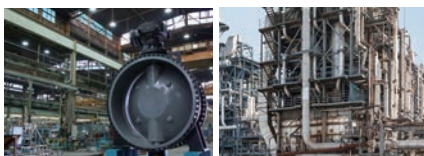
● Valves ● Materials (cracking tubes)
