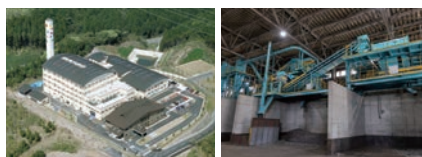
● Waste incineration and melting plants ● Recycling plants
