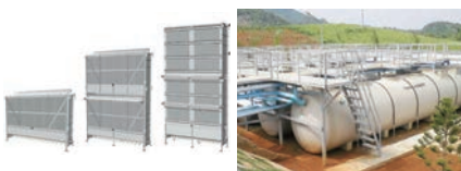
● Submerged membranes ● Wastewater treatment plant (Johkasou)
