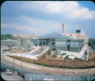
WASTE RECYCLING PLANT
