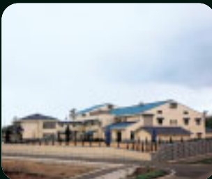
NIGHT-SOIL TREATMENT PLANT
