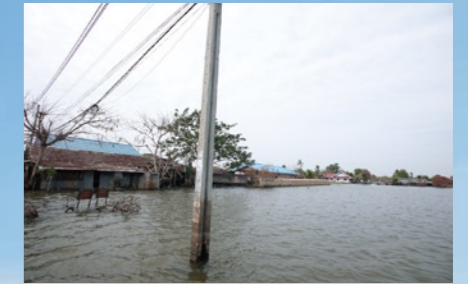
Houses and utility poles hit by flooding (Sai Noi, Nonthaburi Province)
