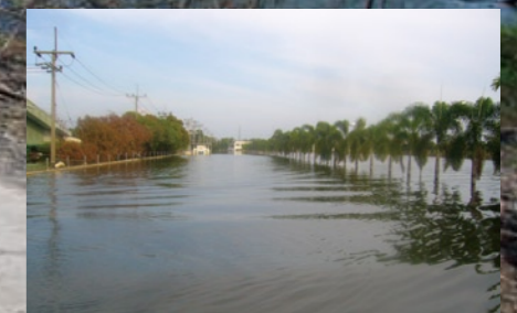
Water purification plant at the Nava Nakorn Industrial Estate at the time of flooding
