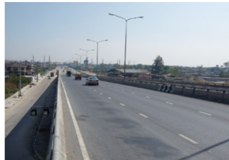
Highways also serve as levees against floods. The current King’s Dike comprises paved roads and riverbanks. (near Lak Hok, Pathum Thani Province)
